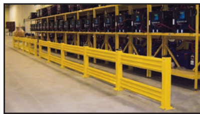
Guarding Battery Racks
